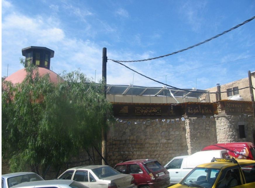
Fig. 10 Solar energy installation on the roof
