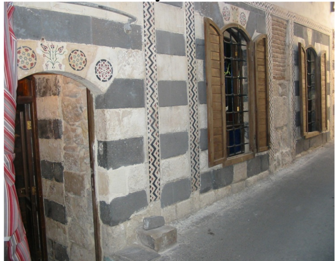
Fig. 6 Main Façade, revealing ornaments
