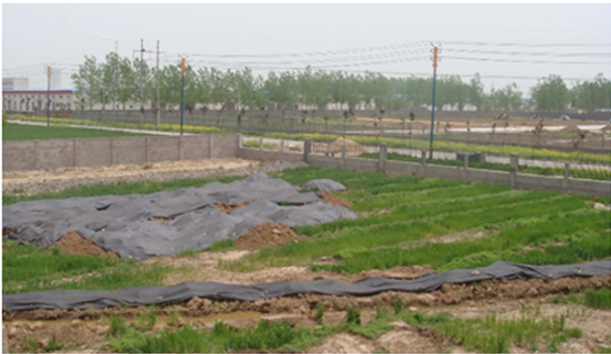
Figure 4: Temporary Cover at Fill Bank
