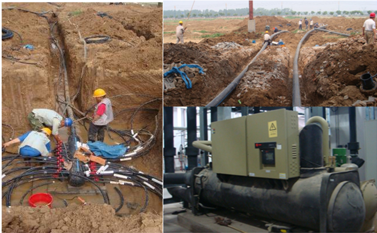
Figure 3: Ground Source Heat Pump (installation)
